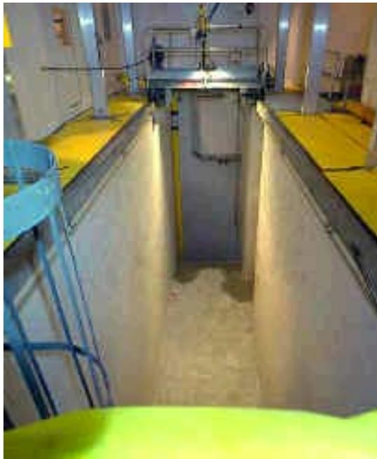
The spent fuel pool emptied of its water in January 1998. The pool contained 68,000 gallons of water up to 30 feet deep for cooling and shielding radioactive fuel and other components.
