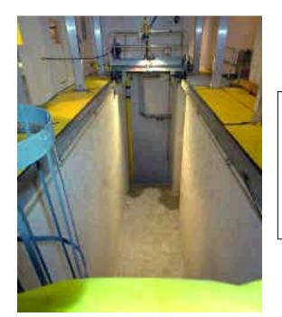
The spent fuel pool emptied of its water in January 1998. The pool contained 68,000 gallons of water up to 30 feet deep for cooling and shielding radioactive fuel and other components.
